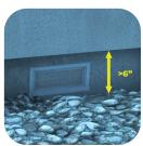
Create 6 inches of vertical clearance between the ground and structure siding
